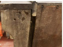
The back bottom brace appears to have come loose. Screws used in repair indicate 1880-1900 for this repair.
